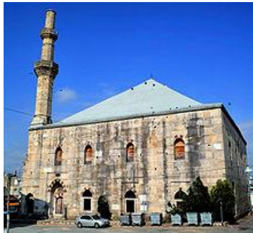
(Pl.15). the gable roof of Mehmet Çelebi mosque, Didymoteicho (1420), (Bourskar,2008).
