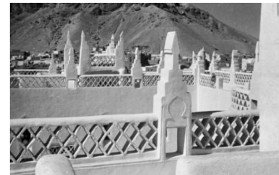
Fig 30. General view of the crenellations “ Tashrīfāt ” atop the buildings in Say‘ūn , by Wilfred Thesiger in 1947. Source: Pitt Rivers Museum, University of Oxford.
