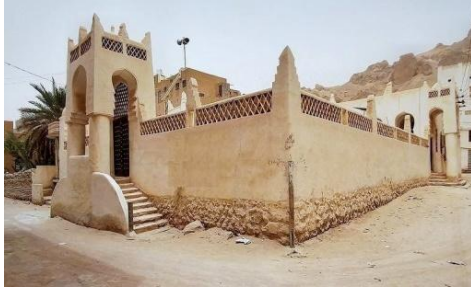
Fig 33. General view of the Mosque of al-Wa‘l in Tarīm.
