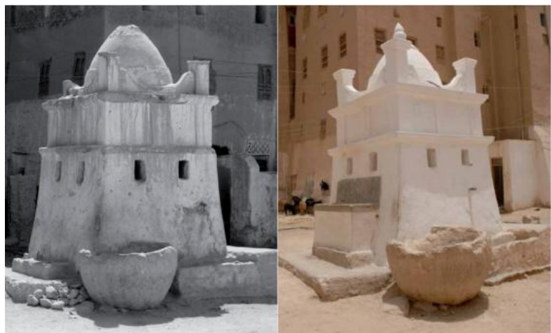
Fig 10. General view of the saqqāyah of the Great Mosque in Shibām, Ḥaḍramūt, before and after restoration in 2003. Source: Damluji, Urban Development Project Shibam, Yemen, On Site Review Report, 2007
