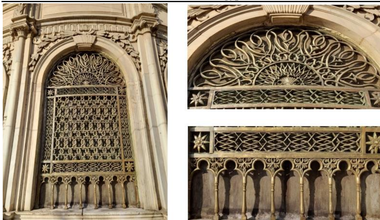
Fig. 13. shows the window grille after cleaning and protection.
