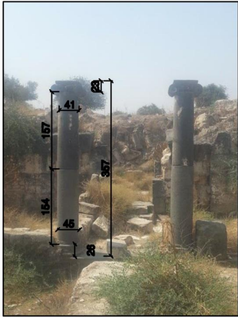
The ratio between the diameter of the column and its height in the building near the forum is 1/8
